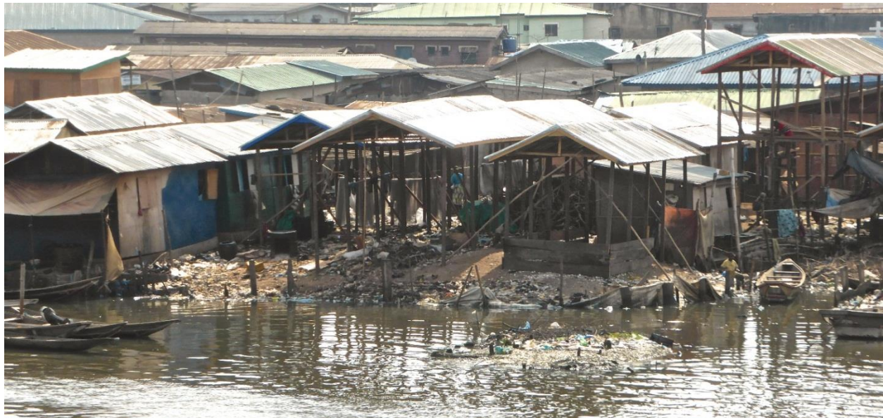
FIGURE 3.7: CONSTRUCTION OF SHELTER AT THE WATER’S EDGE, MAKOKO IN LAGOS
